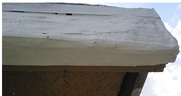
Figure 5: Voila! “Repairs” made. White goop spread over rotten wood. Very much SOP around these parts. (Update: 6-8-23. Further repairs made since then).
