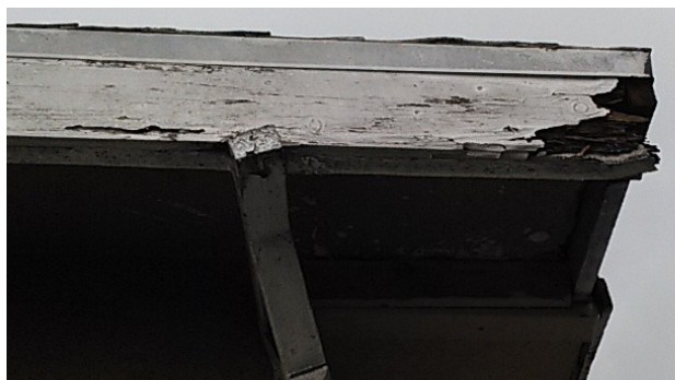
Figure 4: Termite damage, before “repairs.”
